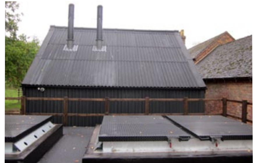
Above Energy Centre and the completed fuel stores
